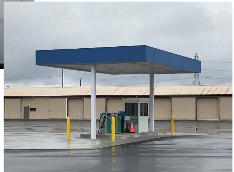
New fueling station canopy
