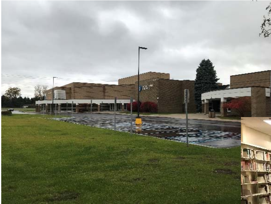
Parking lot repaving
