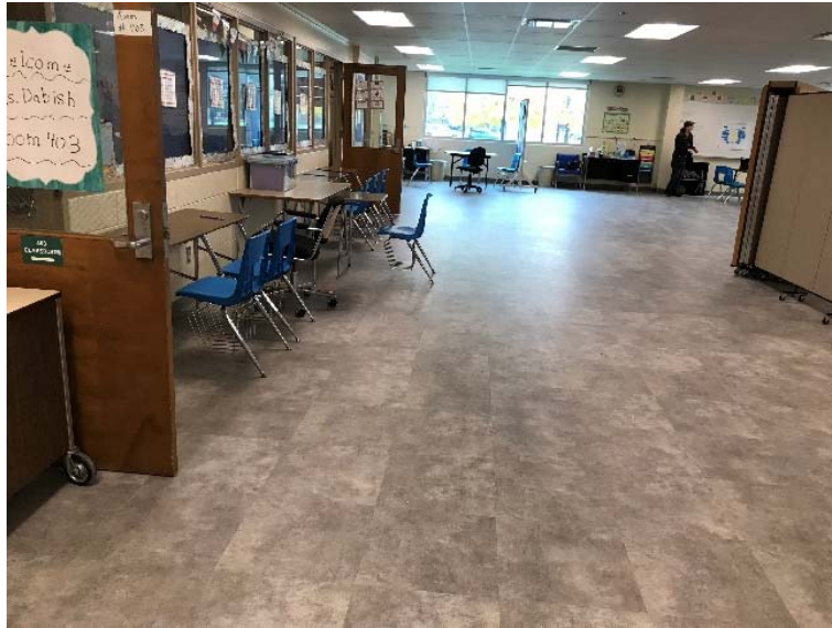
New door hardware and emergency lights
