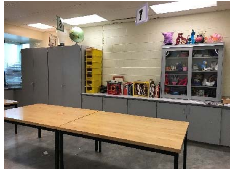
New classroom flooring and casework
